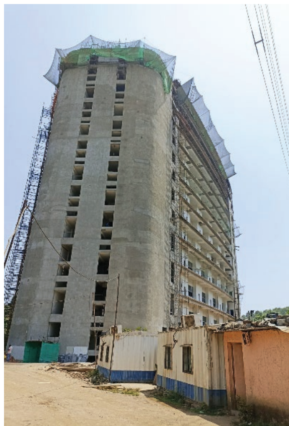
Upcoming Research Park Building as on April 2022
