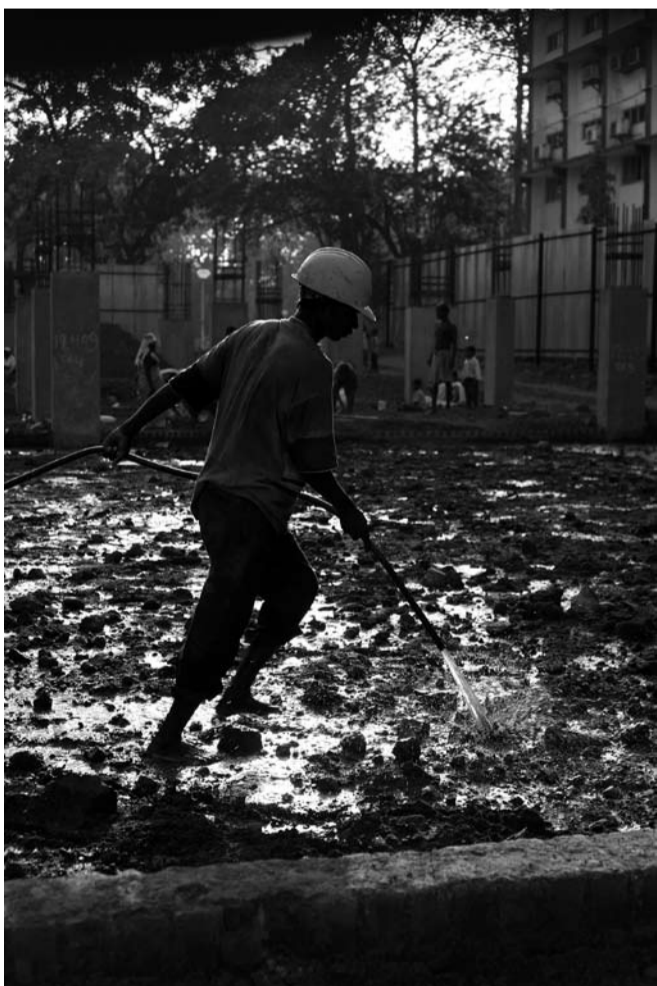
Grace and rhythm lie waiting to be captured in the most humdrum of tasks, as our cameraman discovers. Here, the soil is being loosened with jets of water before it is dug up.
